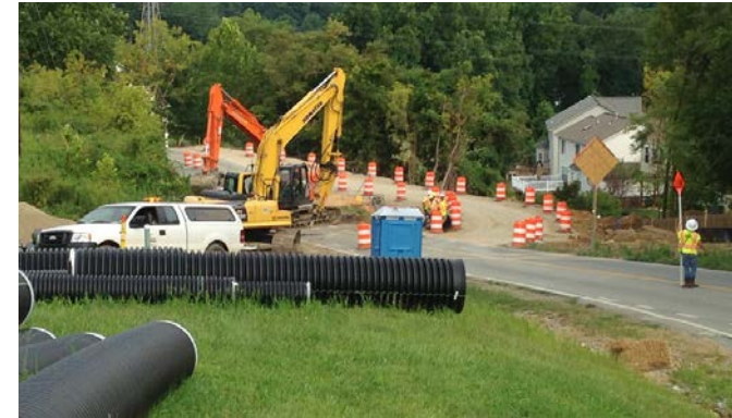
Cotton Hill Road Under Construction
