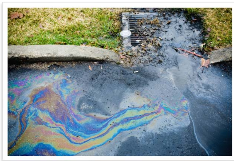
An illicit discharge of oil into the storm drainage system.
