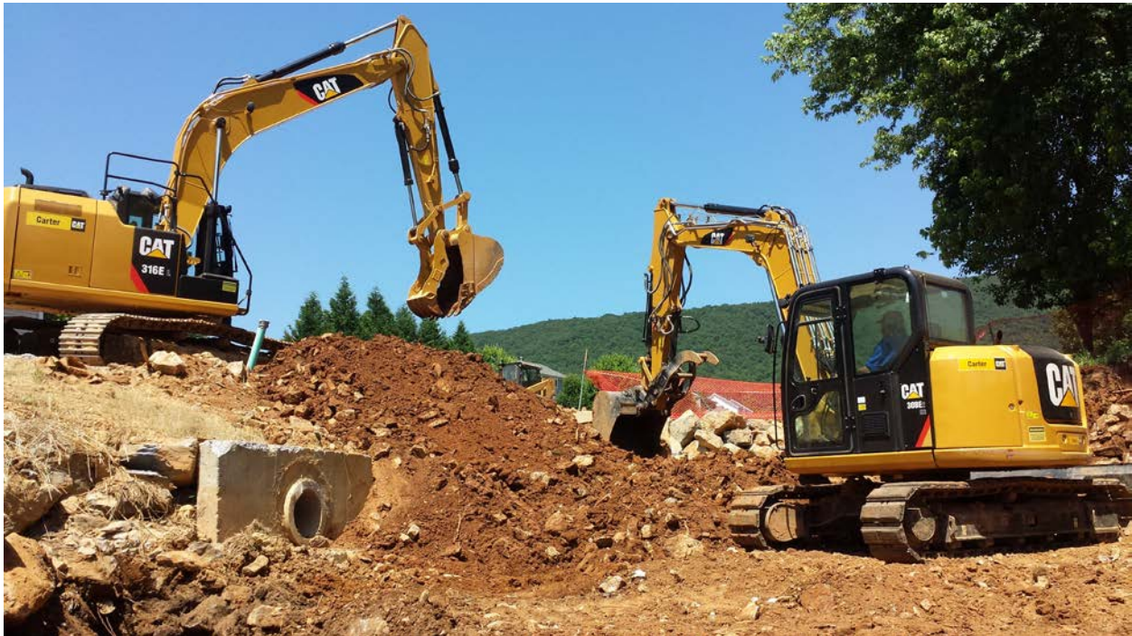
County drainage crew improving an existing storm drainage system.
