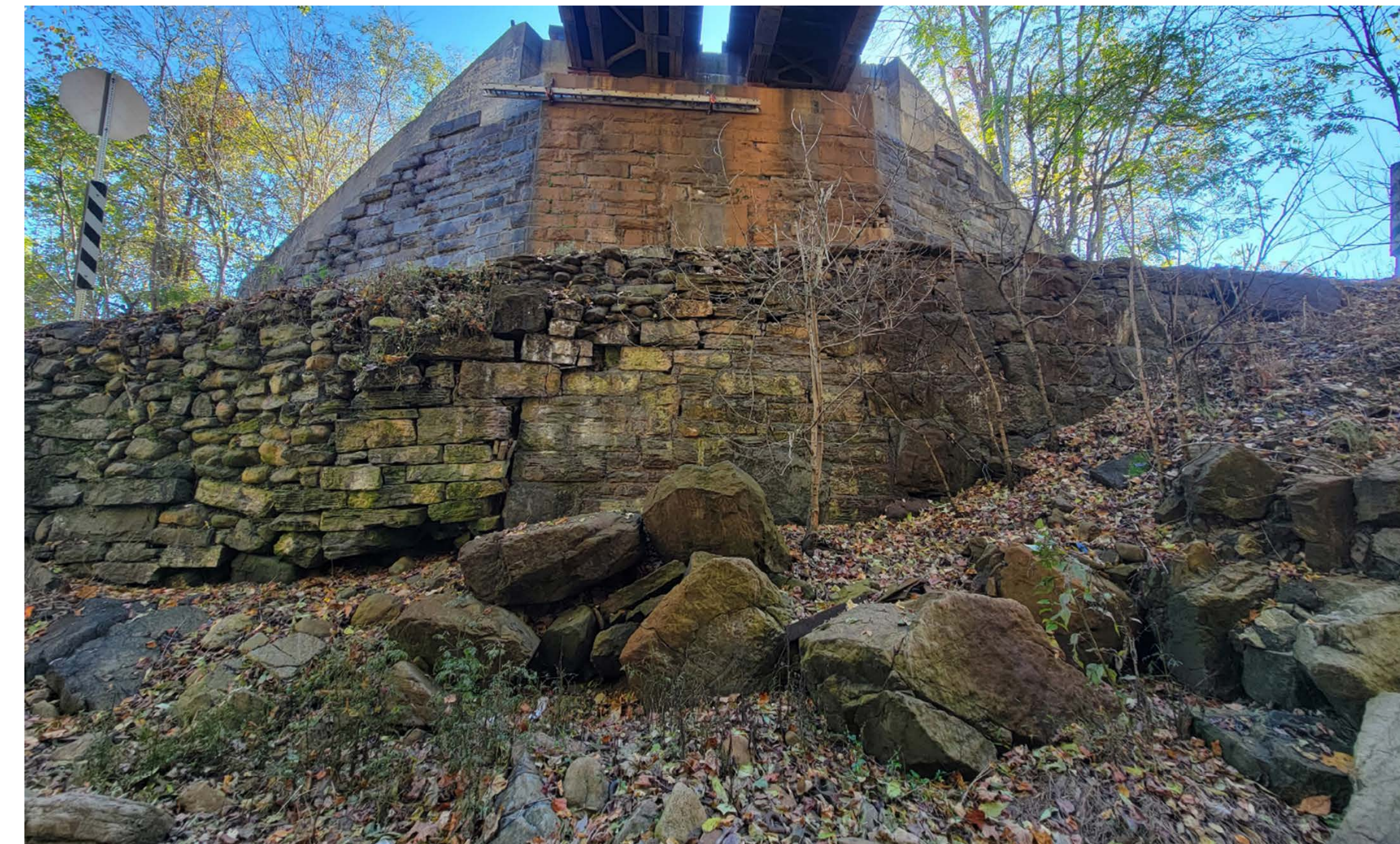
Existing Rock Retaining Wall between Roadway and Creek
