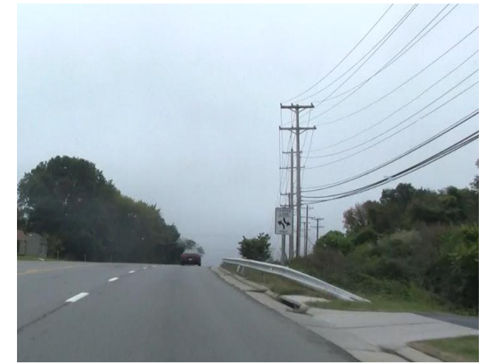
Photograph 5.35 – Out of Compliance Guardrail End Treatment
