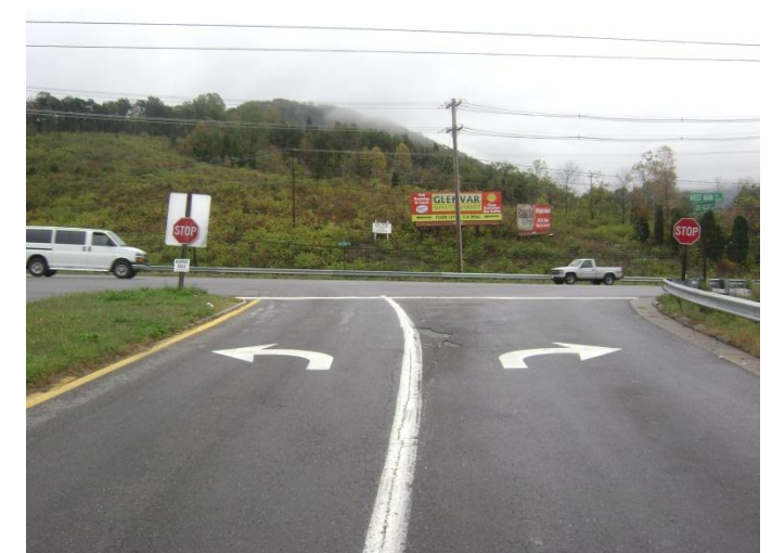
Photograph 5.4 – Dow Hollow Rd Southbound Approach – No Route Signs Provides on Far Side of Intersection
