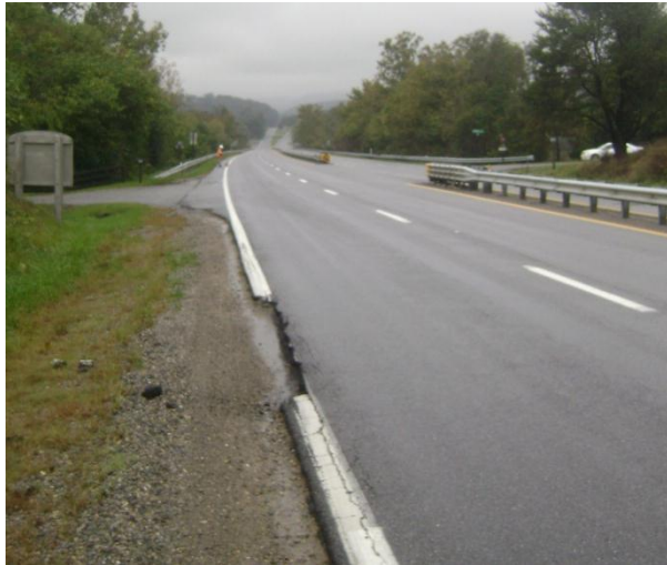
Photograph 5.36 – Edge Drop Off Along Route 11/460
