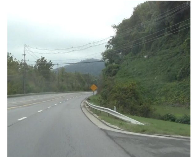
Photograph 5.25 – Out of Compliance Guardrail End Treatment
