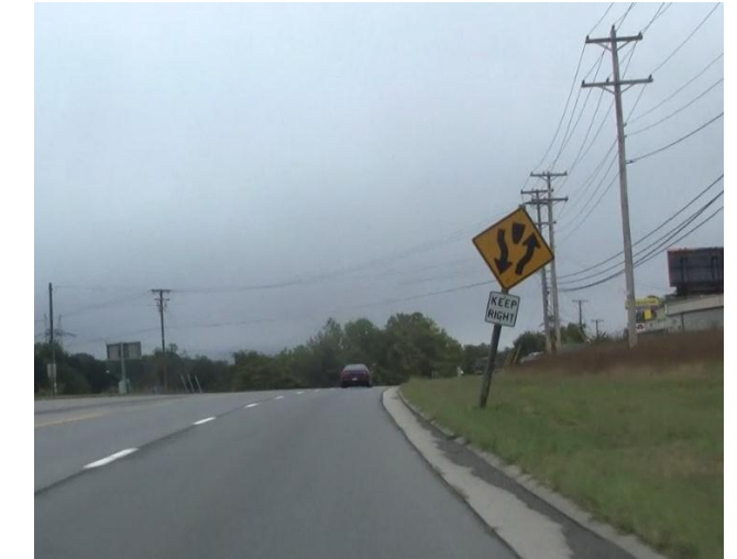
Photograph 5.17 – Leaning “DIVIDED HIGHWAY” and “KEEP RIGHT” sign
