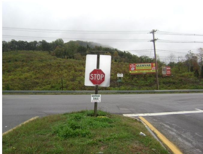
Photograph 5.5 – Dow Hollow Rd Southbound Approach – Stop Sign Mounted Behind Larger Sign
