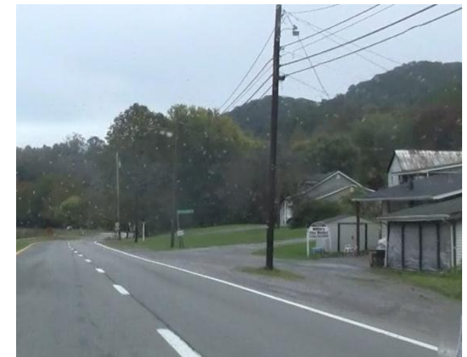
Photograph 5.21 – Example of Access Along the Route 11/460 Corridor with a Wide Throat/Wipe Down Entrance
