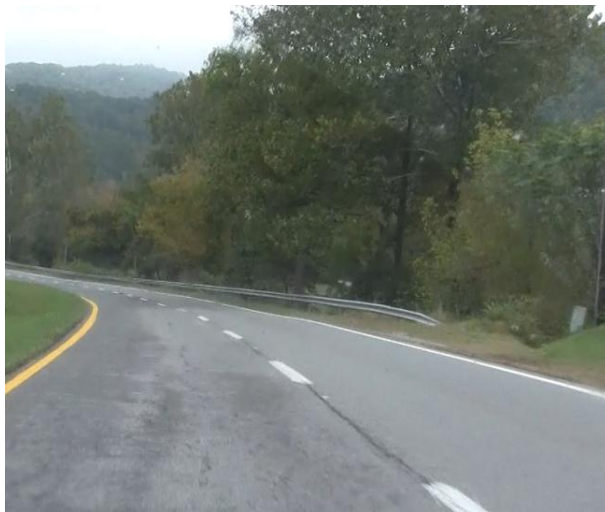
Photograph 5.30 – Out of Compliance Guardrail End Treatment
