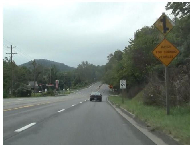
Photograph 5.19 – Route 11/460 Approach to West River Road – Faded Advanced Warning Signs
