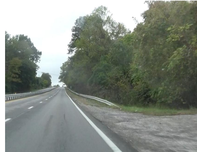
Photograph 5.24 – Out of Compliance Guardrail End Treatment
