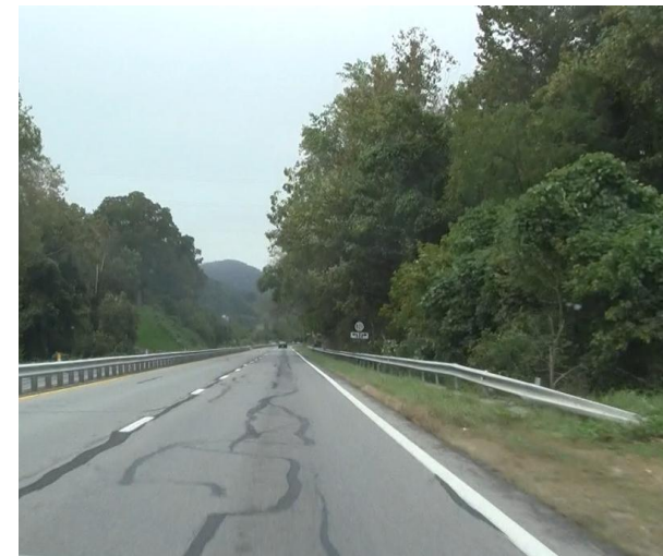
Photograph 5.26 – Out of Compliance Guardrail End Treatment
