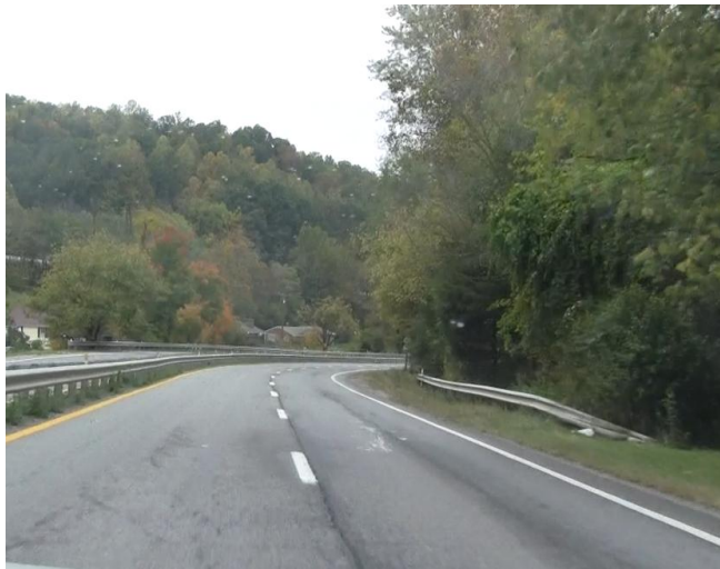
Photograph 5.28 – Out of Compliance Guardrail End Treatment
