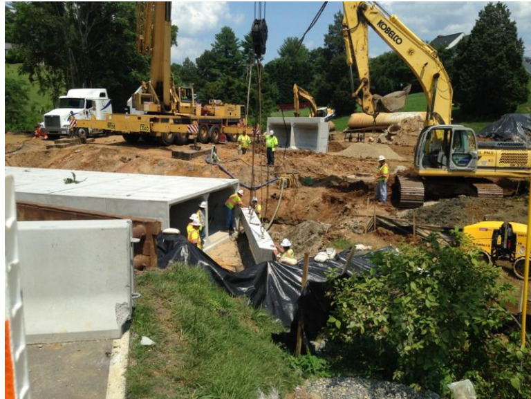
Drainage Improvements Under Construction
