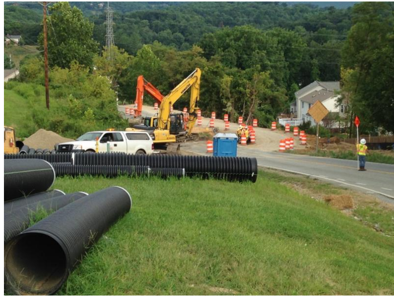
Cotton Hill Road Under Construction
