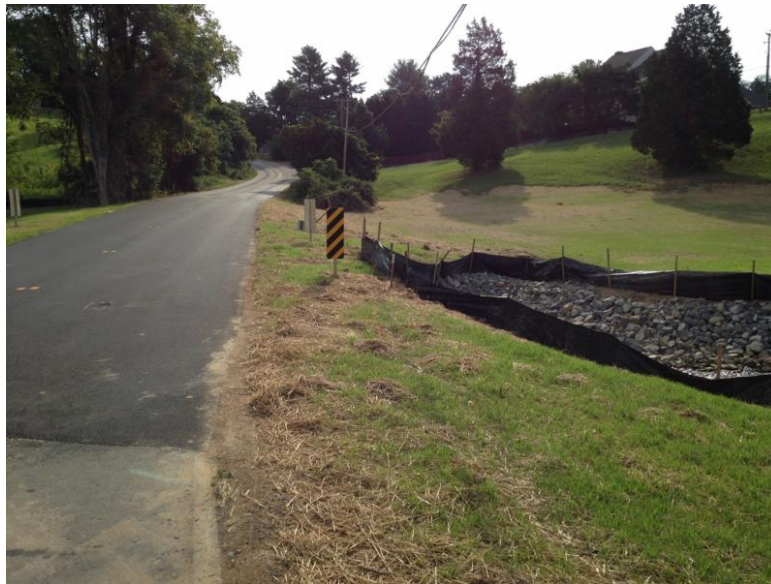
Drainage Improvements Completed
