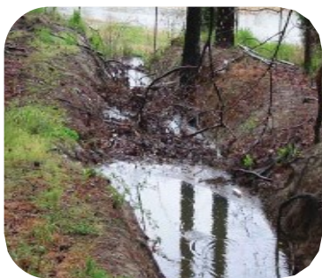
Tree branches and leaves dumped by homeowners are a common cause of storm drain blockages that contribute to flooding during heavy rains.
