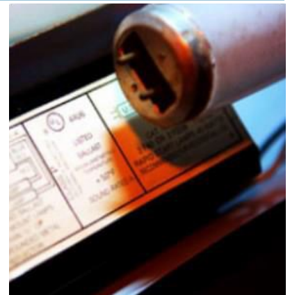
Older Fluorescent light ballasts (FLBs) can contain PCBs. Because of this, FLBs should be removed and disposed of by trained professionals.
