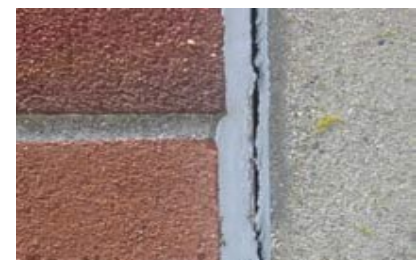
Old paint and caulk and nearby substrate (brick, masonry, cinder block, wood, etc.) may contain PCBs. Care must be taken during removal of these materials to avoid the creation of dust and to contain contaminated waste.
