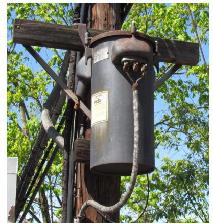
Transformers containing PCBs , which contain more than 50 ppm of PCBs, are subject to specific EPA regulations. Proper PCBs identification labels must be visible near the access and on the transformer itself.
