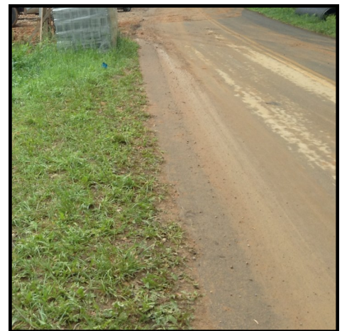
MS-17 Violations: Sediment tracking onto paved surfaces; sweeping is required at the end of each day, at a minimum.
