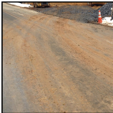
MS-17 Violations: Sediment tracking onto paved surfaces; sweeping is required at the end of each day, at a minimum.
