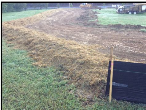
MS-4: Stabilized perimeter dike
