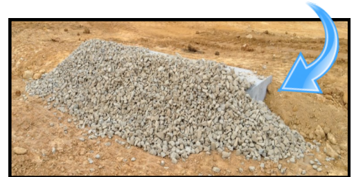
MS-10: Proper inlet protection for a curb inlet
