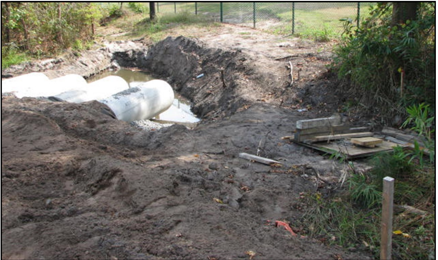
MS-19 Violation: Inadequate channel at point of discharge; bed and banks will erode; banks will overtop.
