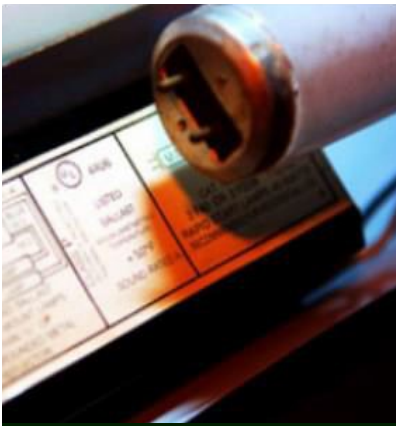
Older Fluorescent light ballasts (FLBs) can contain PCBs. Because of this, FLBs should be removed and disposed of by trained professionals.
