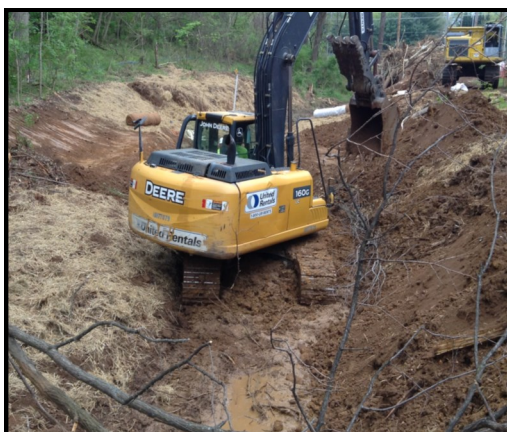
MS-12: Working in a live watercourse; once complete, temporary or permanent channel lining will be applied per MS-11
