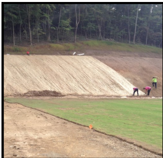
MS-7: Minimizing erosion of slope face using fabric
