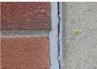
Old paint and caulk and nearby substrate (brick, masonry, cinder block, wood, etc.) may contain PCBs. Care must be taken during removal of these materials to avoid the creation of dust and to contain contaminated waste.
