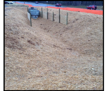
MS-6: Stabilized sediment trap
