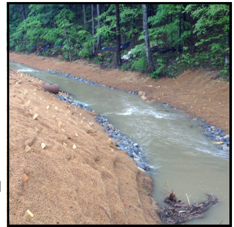
MS-15: Stabilized stream bed and banks
