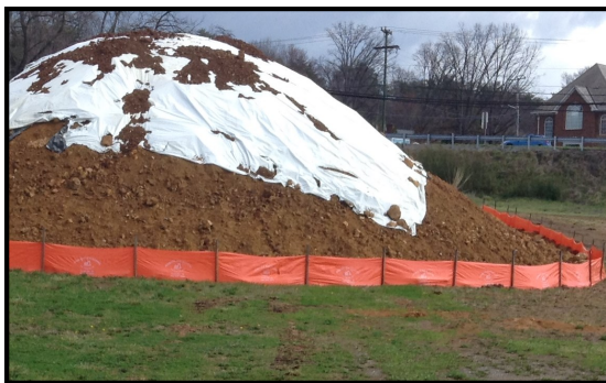
MS-2: Stabilized/protected soil stockpile
