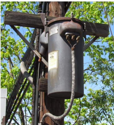
Transformers containing PCBs , which contain more than 50 ppm of PCBs, are subject to specific EPA regulations. Proper PCBs identification labels must be visible near the access and on the transformer itself.
