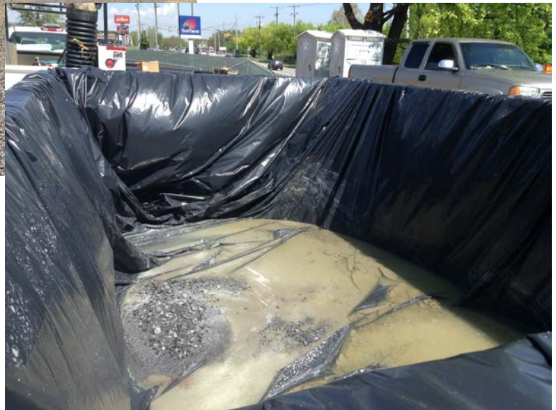
Concrete washout facility at LewisGale Emergency Center project
